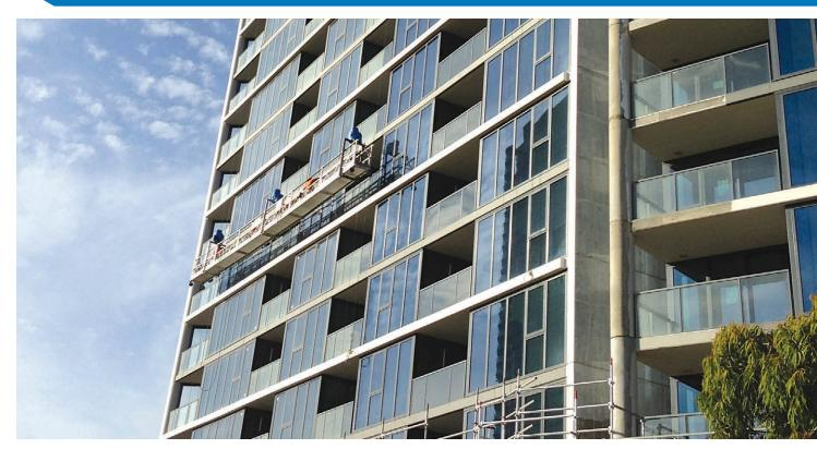
Swing stage scaffolds take men, tools and materials up to the ideal working height to get the job done correctly and efficiently. They are the ideal working platform in almost every area of construction and maintenance involving a vast range of trades because of their versatility. All Systems modular swing stage scaffolding can be designed in any configuration up to 16mts in length.
